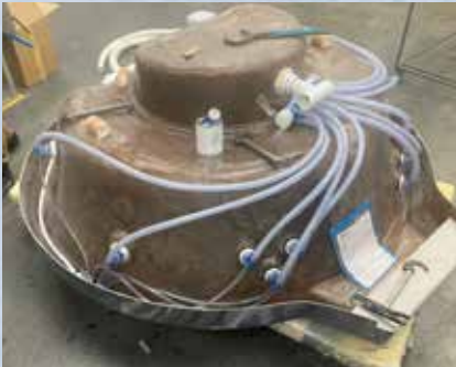
FIGURE A: Spillover side left/left side if viewing from back of standard spa: water lines and air lines (clear) connect to the canister (top) and jet bodies.
