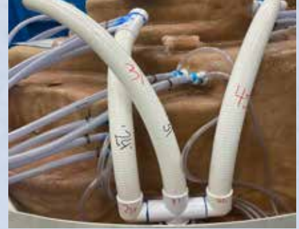
FIGURE C: Diverter Valve connection to regulate the jets to eurojets. (feature of 25 jet models only)
