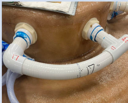
FIGURE D: Diverter Valve connection to regulate the jets to eurojets. (feature of 25 jet models only)
